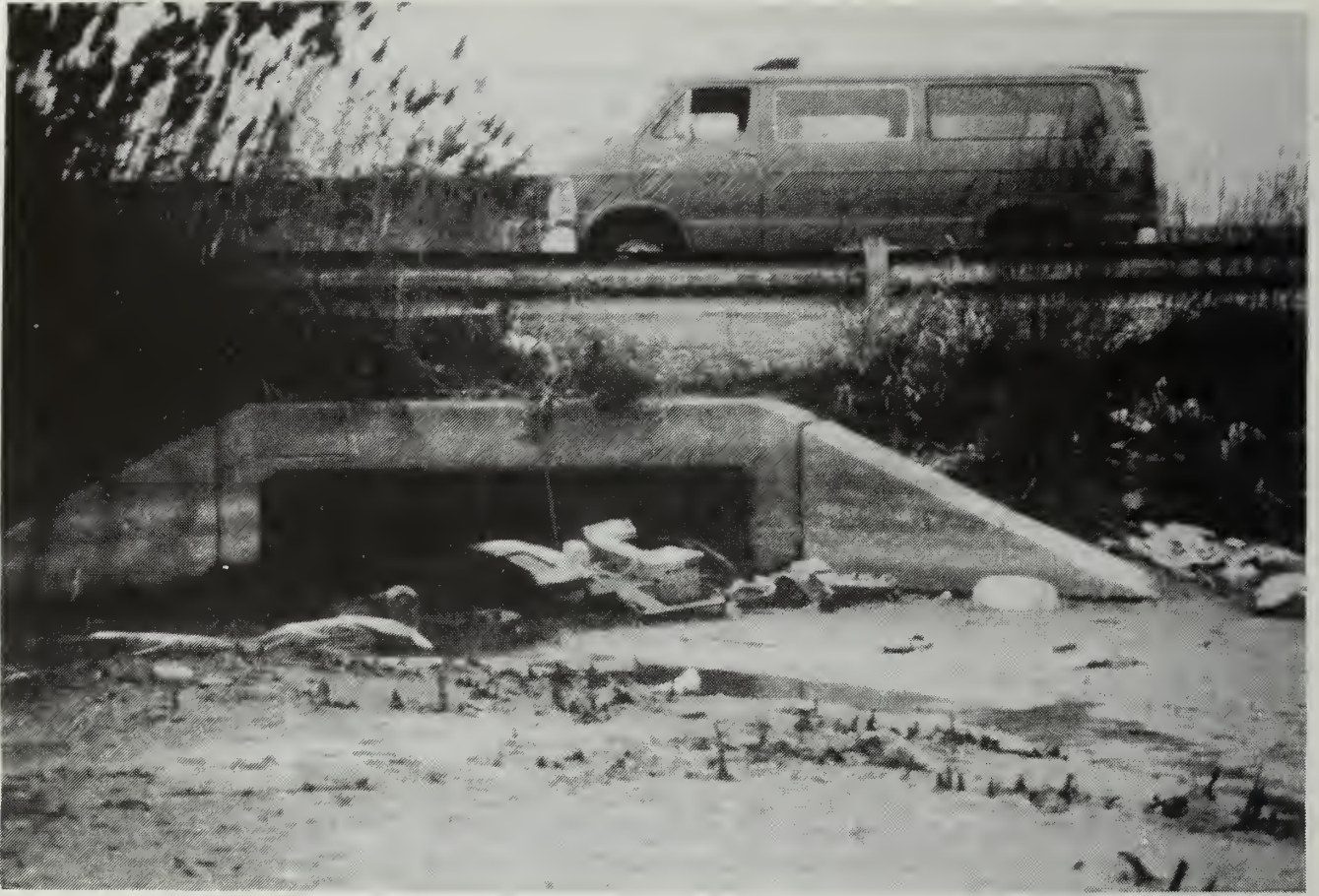
Drainage outlet from Interstate 94. In an FY'89 study, Dr. Nani Bhowmik and William Fitzpatrick of the State Water Survey found that drainage from I-94 and adjacent landfills and roads was the largest measured source of arsenic, lead, and chromium to Lake Calumet--over 4 pounds per hour on one day during a rain storm.
